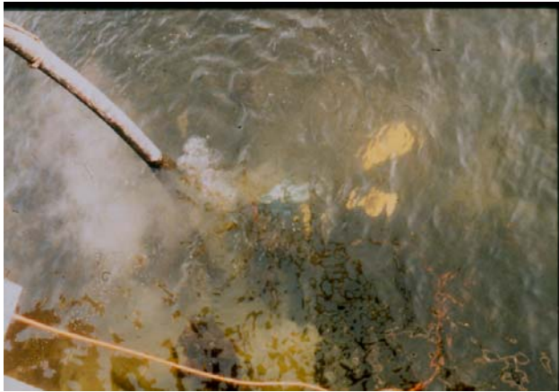
Pumping concrete with and without an underwater concrete admixture.
